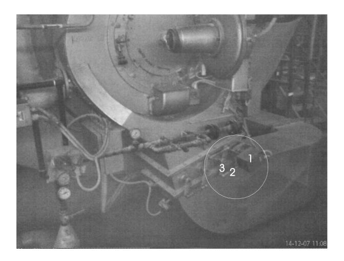
The ideal solution where to remove the servomotor and refit it on a console on top of the air channel say 50 cm right of the first shaft. The actuator should then turn the first shaft over a new link connection with two new arms. The new arm on the first shaft should then include the sledge part of the trim actuator and the electrical part on a console again on console on top of the flue channel.
