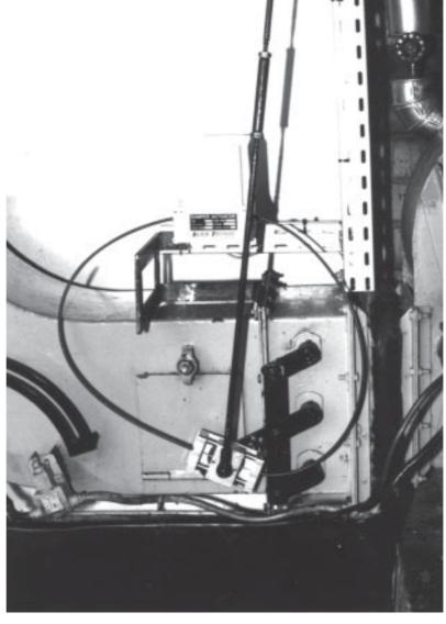
The fotograph show a position near to minimum air position (she sledge is near to a 90 ° angle to the linking rood and when this and the arm is moved upwards the the angle gets smaller and smaller until the sledge is moving in exact in the same rirection as the linking rod adding a trim action of  $\pm$  25 mm to the original air/fuel ration.
