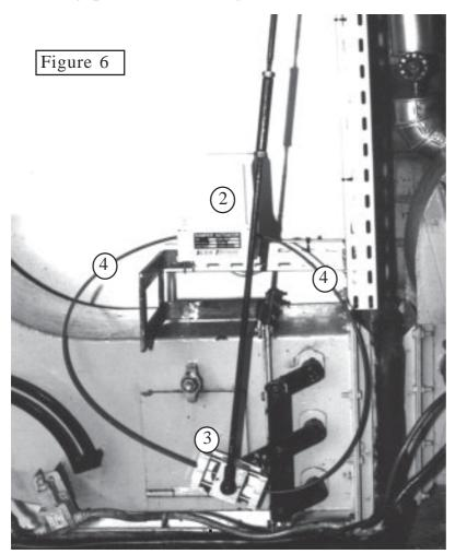
transferred by two cables (4). This way the system can easily be adjusted to modify the air rate  $\pm 15$  % all over the modulation range of the burner - giving a good safe regulation.
